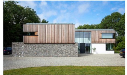
The flint wall reflects the local soil. The white brickwork acts as a foil to the larch cladding DAVID GILES
