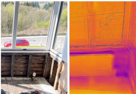
Using a thermal camera, Mick Wall discovered that underneath the bay window there was nothing at all between the internal plasterboard and the outside tiles
