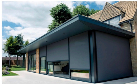
External shutters can be used to block the sun’s heat, such as those seen here from Caribbean Blinds JAHED QUDDUS
