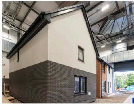
The Energy House 2.0
